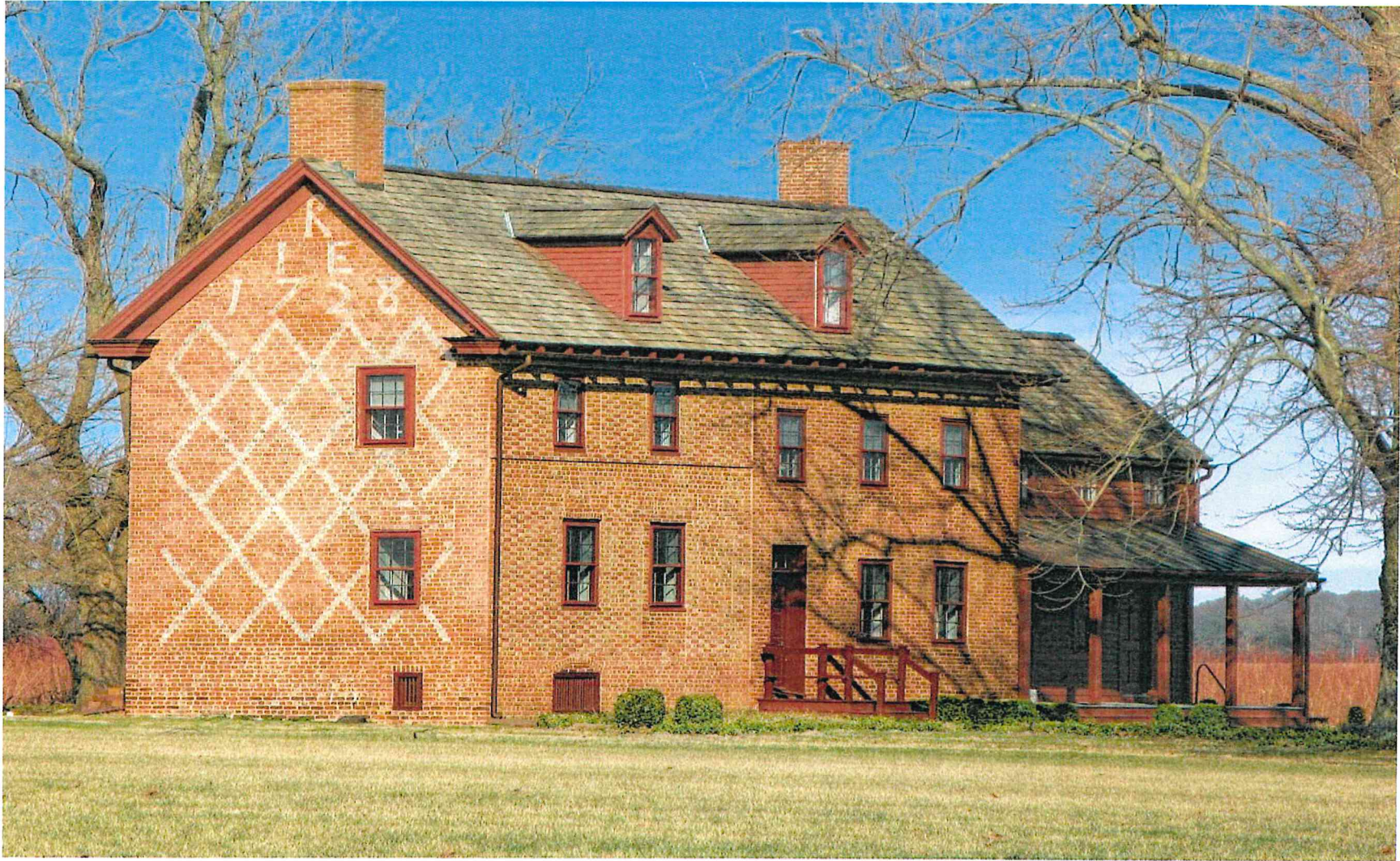
John Remington House (1728). This private home was owned by John and Elizabeth Remington and located on Roadstown Road, Cumberland County. This Delaware Valley patterned end brick house was built in the Federal style of architecture with Flemish influences. These homes were built by and owned by the Quakers and this type of architecture is unique to old “Western New Jersey” now called southern New Jersey.
